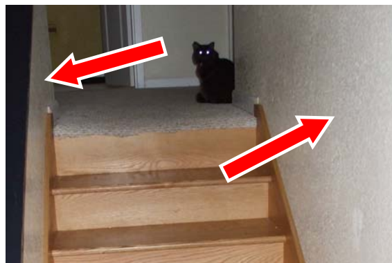
Handrail missing
