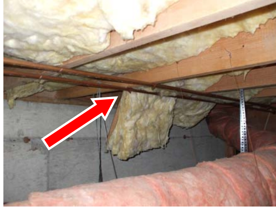
Un-insulated domestic water pipes
